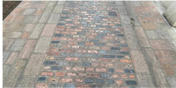
Granite setts with a high concentration of blue indicate vehicle access through this heritage setting. Joints have been over-filled to improve pedestrian accessibility.
