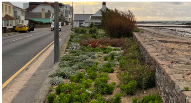
The purposing of part of the seawall along Havre des Pas has allowed for a well-executed, sensitively-designed planter/parklet.
