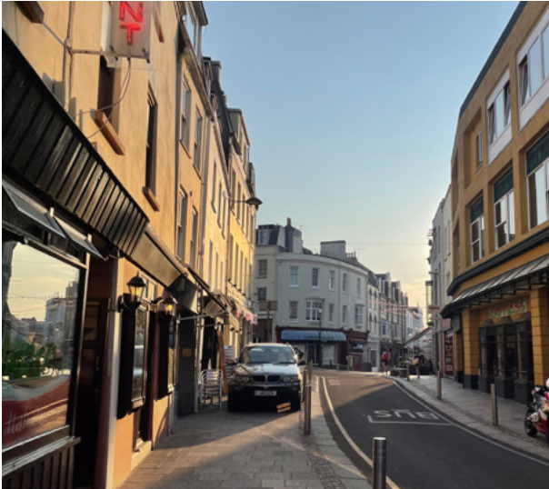
Grand townhouses and buildings of a consistent, 4-storey scale bring a uniformity along La Motte St. Neat shop frontages enhance character.
